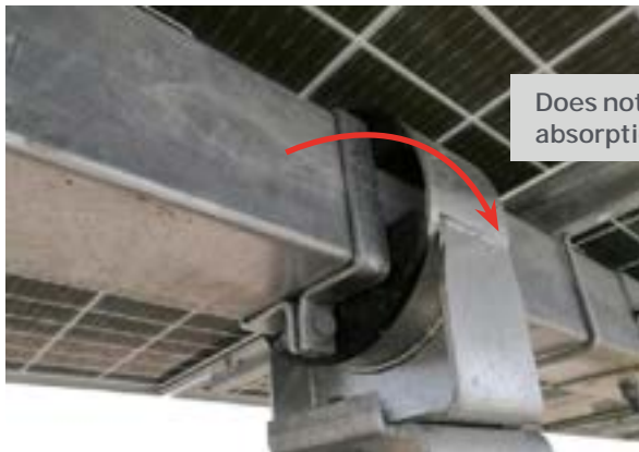
Image 16: Cylindrical bearing structure
